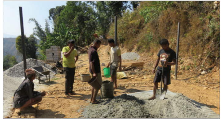
Local volunteers in Sipapokhare village laying the foundation for a home
