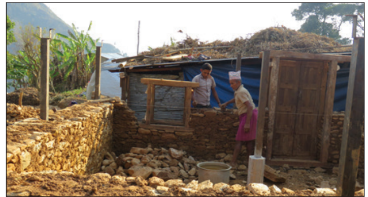
A man and his son rebuilding their home with clay and stones
